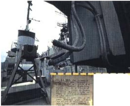
The Eldridge: Power-cables from the Phil. experiment are still visible 50 years later.
